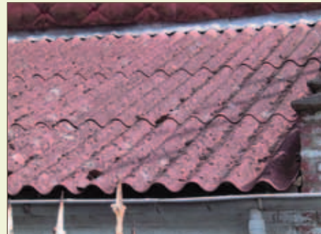
Dakgolfplaten in asbestcement
